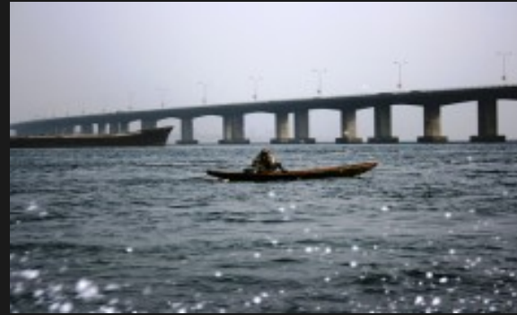
3 rd Mainland Bridge
